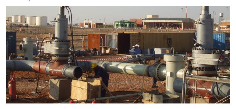
Our range of specialist hot tapping equipment allows a connection to be made to a piping system or a vessel (onshore or subsea), **without shutdown or interruption to production**. Our services can also perform a temporary intervention and isolation of the pipeline while it is operational (therefore avoiding downtime), to provide rectification to the pipeline or to restore integrity of the system.
