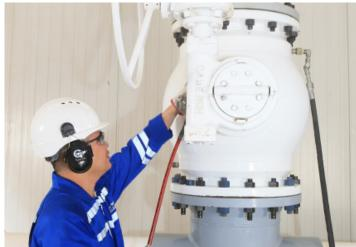
Maintaining the integrity of the valve assembly is crucial for continuous operation of assets. We understand the importance and hence have applied our knowledge and experience to develop a robust and proven method of flushing and lubricating valves on-line; without having to close the valve.
