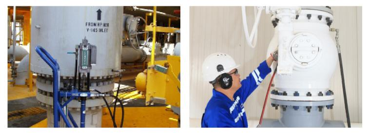
Maintaining the integrity of the valve assembly is crucial for continuous operation of assets. We understand the importance and hence have applied our knowledge and experience to develop a robust and proven method of flushing and lubricating valves on-line; without having to close the valve.
