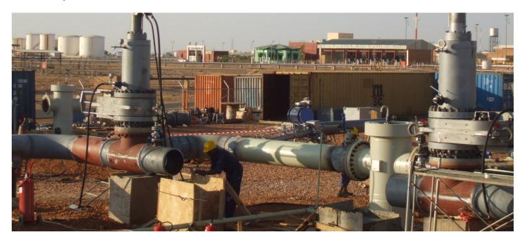
Our range of specialist hot tapping equipment allows a connection to be made to a piping system or a vessel (onshore or subsea), without shutdown or interruption to production. Our services can also perform a temporary intervention and isolation of the pipeline while it is operational (therefore avoiding downtime), to provide rectification to the pipeline or to restore integrity of the system.
